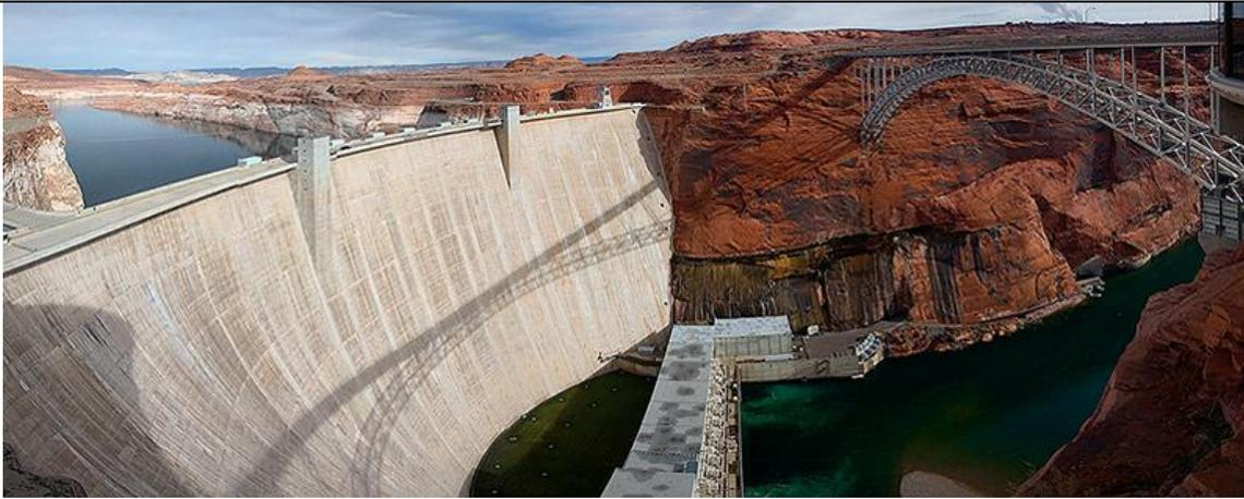
**Concrete arch-gravity dam: Glen Canyon Dam on the Colorado River in Arizona, USA**
