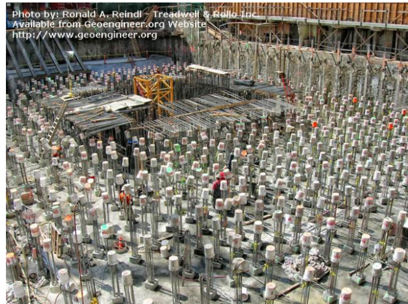
Mission Piles, San Francisco, CA. After the 900+ piles had been driven for the 60-story high-rise.
