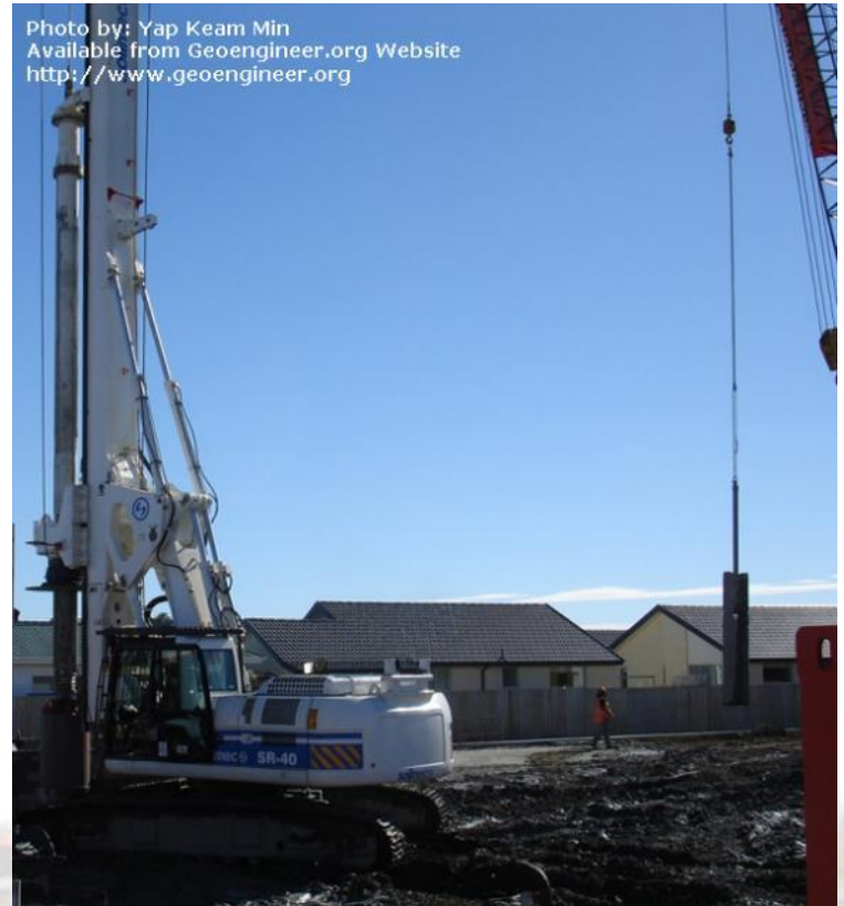
Bored piling in New Zealand
