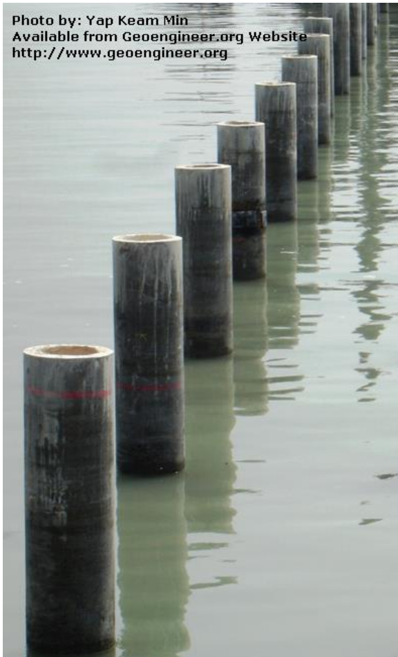
Precast spun prestressed concrete piles used in marine condition.
