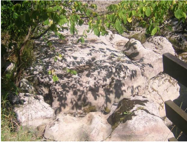
Figure 20. Joints widened by solution in Caldbeck river bed.
