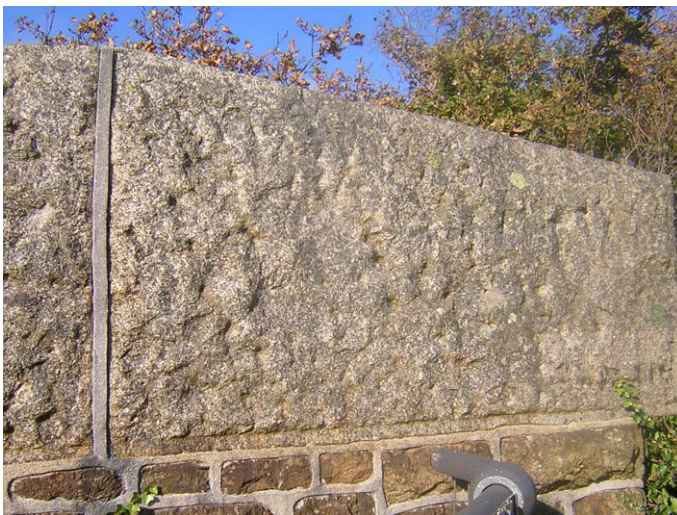
Figure 15. The granite capstone.
