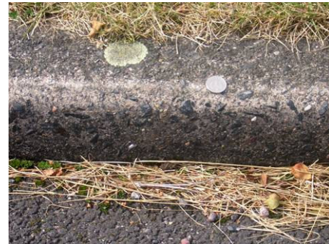
Figure 4. Site 2 West Side Curb.
