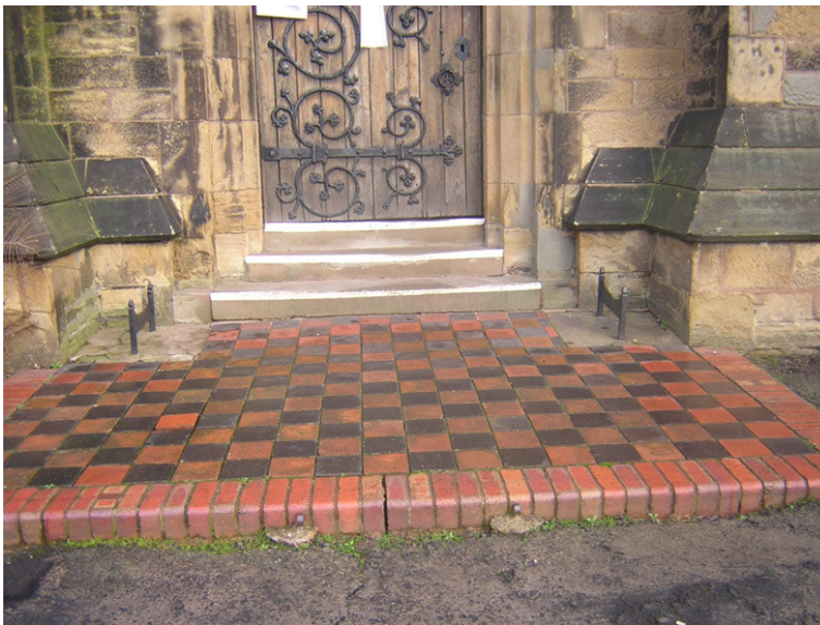
Figure 12. The tiled approach to St Mark’s Church door.
