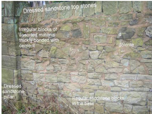
Figure 13. North section of the vicarage wall
