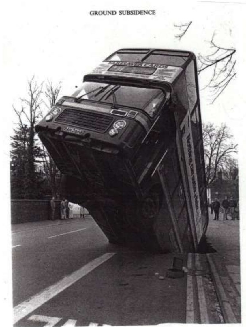
Figure 1.1 A bus caught at an unusual angle when a road collapsed beneath it early in 1988 in the city of Norwich. The subsidence was due to failure of weathered chalk above old abandoned mines (Photo: Eastern Counties Newspapers).
